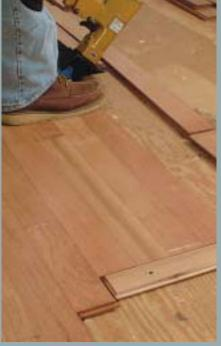
A temporary stop establishes the border's line. Screwed into the subfloor, scrap flooring provides a clean starting point for the flooring and a fast, straight line for one side of the floor's border.
