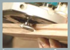
Router cuts new groove to mate floor and border. Using a top-bearing router bit, the author can cut a groove and mate two boards groove to groove with a spline.
