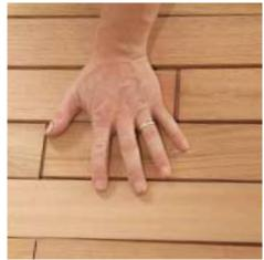
Staggered butt joints make a stronger, better-looking floor. Joints on adjacent rows should be spaced at least 6 in. apart to keep the floor from flexing under load.
