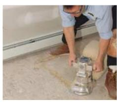
Edging sander makes quick work of the subfloor's high spots. Created by a crowned joist or the joint between plywood sheets, high spots can be sanded down to flatten the subfloor.
