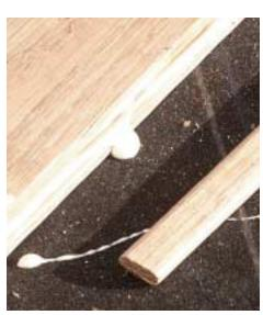
Reverse the flooring's direction with a slip tongue. Lengths of hardwood splines are glued and pinned into the groove of a center starter course. The flooring can then be nailed down in the opposite direction.
