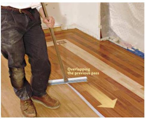
into the air. I also make sure that dust that has collected on windowsills, the floor and other horizontal surfaces is picked up with a clean, lint-free tack rag. To make a tack rag, I lightly dampen a clean rag with the solvent used in the finish (mineral spirits for oilbased finishes, water for water-based finishes) and wrap it around a push broom. Moving the broom in only one direction helps to keep the dust on the rag.
